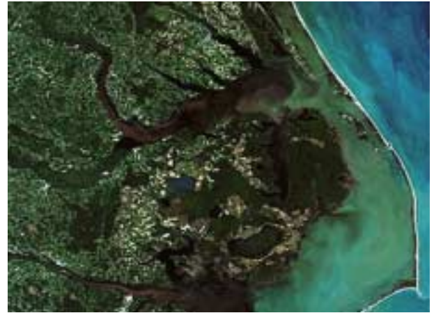
Figure 5.3 North Carolina coast after Hurricane Floyd
