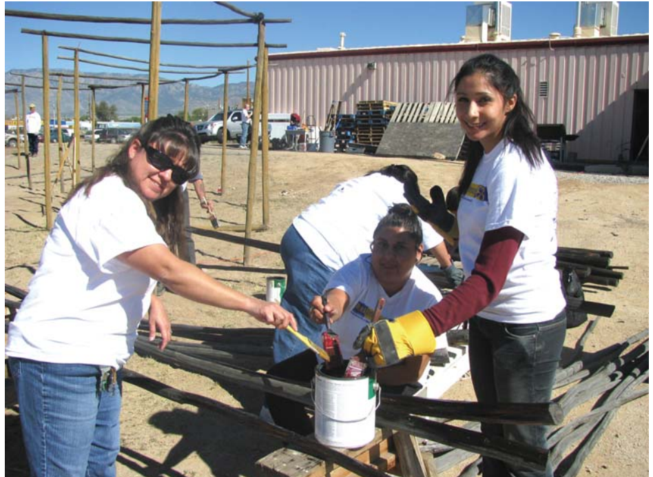
DAY OF CARING: Employees from NNSA's Service Center participate in an annual Day of Caring , volunteering their time at several projects. A project this year included staining a ceremonial site structure at the Albuquerque Indian Center. Helping with this effort are (left to right) Elaine Duran, Denise Trujillo and Emily Sanchez.
