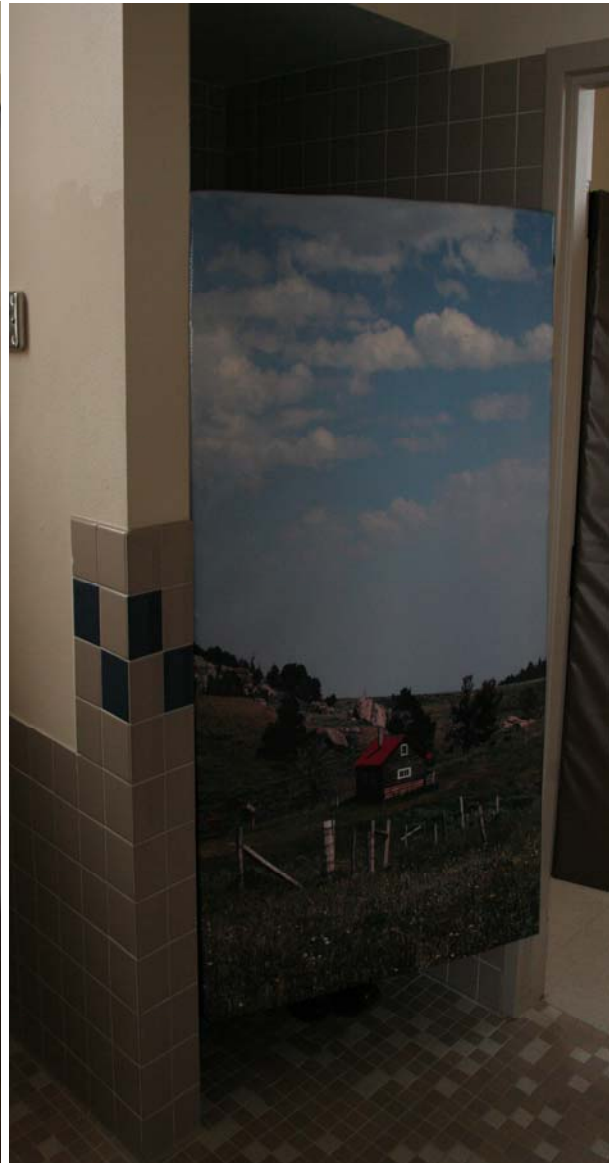
Figure 2: Soft Suicide Prevention Door (SSPD)
