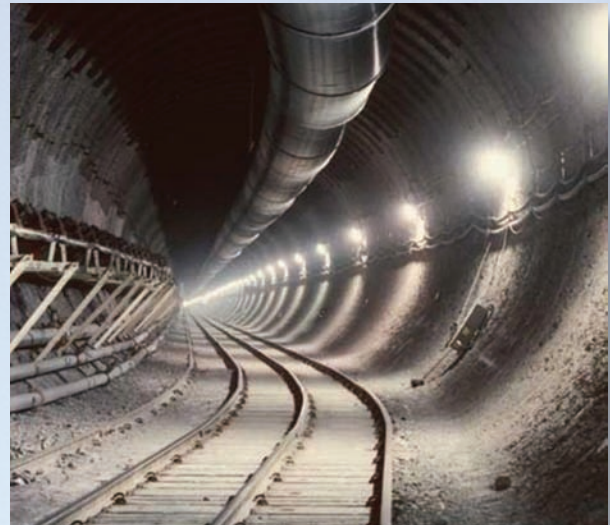
The main tunnel under Yucca Mountain, showing ventilation pipes and train tracks.
