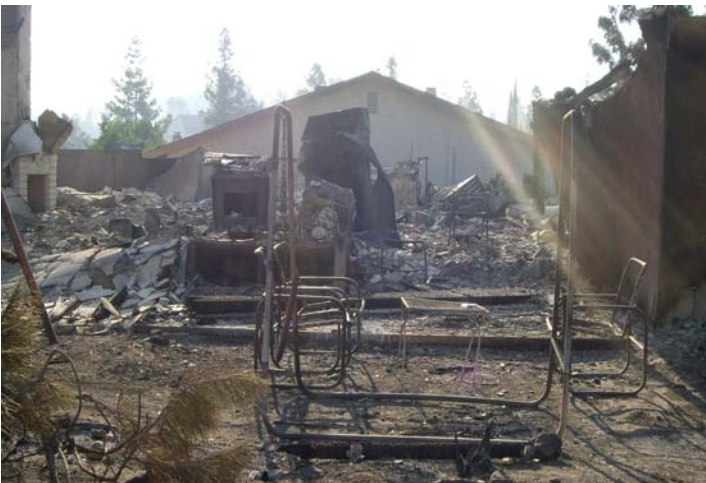
Picture of home in Rancho Bernardo that was completely destroyed by the Witch Fire Storm.
