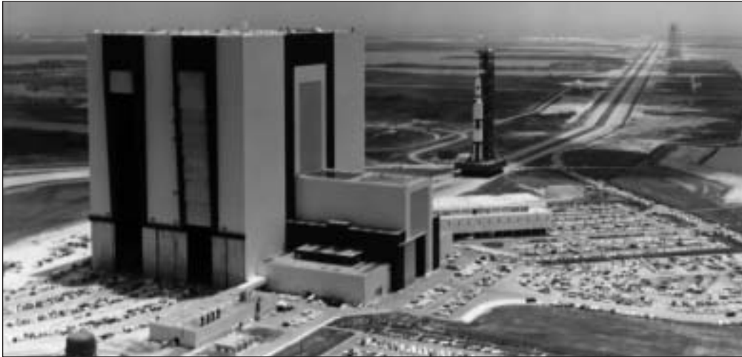
Figure 1-11 The massive size of the Saturn V and the Vertical Assembly Building (later renamed the Vehicle Assembly Building) are shown in this 1969 aerial photograph with the launch complex more than three miles in the background. Delivering 7.5 million pounds of thrust in its first stage and standing 363 feet tall, it was the most powerful rocket ever successfully built and flown with astronauts aboard. (NASA photo)
