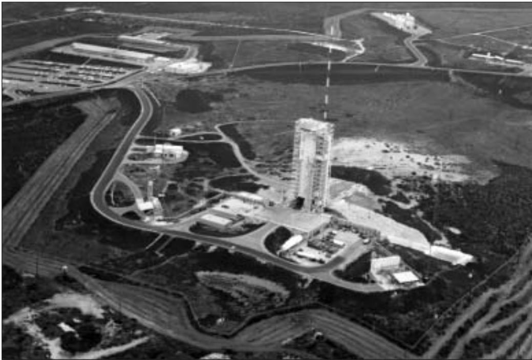
Figure 3-5. This is an aerial view of Space Launch Complex (SLC)-4 at Vandenberg Air Force Base, a site used to launch Titan IIIB rockets. (U.S. Air Force photo)
