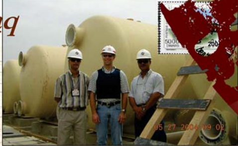
Paul Kerl, normally a Project Manager from the Los Angeles District, is currently serving as the Lead Project Manager for the USAID Project Office in Baghdad, Iraq. He is shown here (center) discussing construction progress with Iraqi engineers on 50 pressurized sand filters at Iraq's largest water treatment plant. (Photos provided by Paul Kerl)
