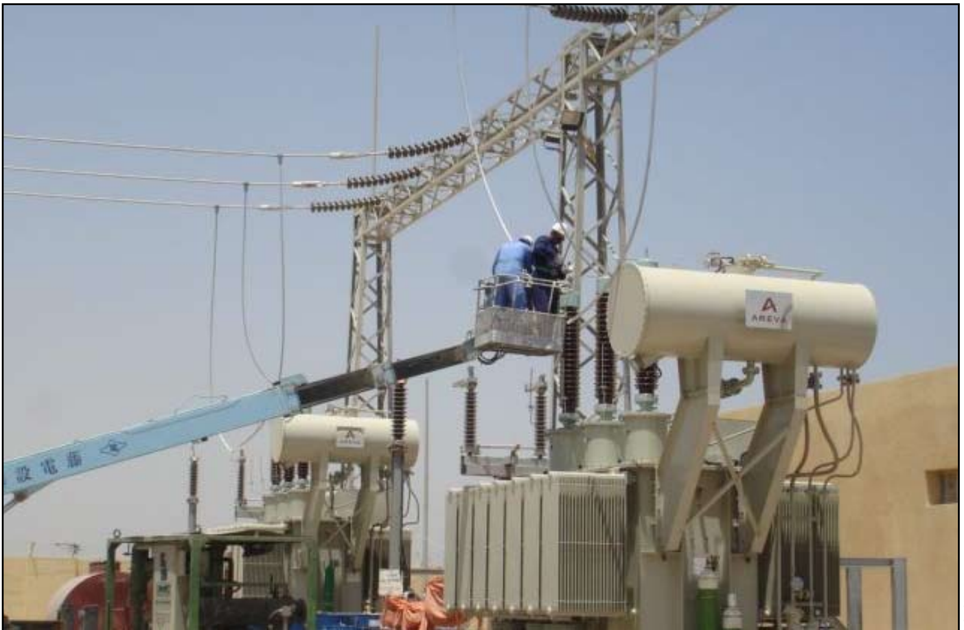
Iraqi workers prepare to connect power cables to one of the transformers at Al-Garma substation. The 132kV substation will enhance the quantity and reliability of power to Gas/Oil Separation Plants and residents in the region.
