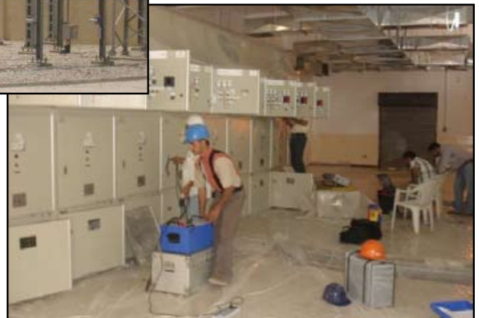
Below: Iraqi workers and engineers prepare to test the electrical system at the high voltage switch gear room.
