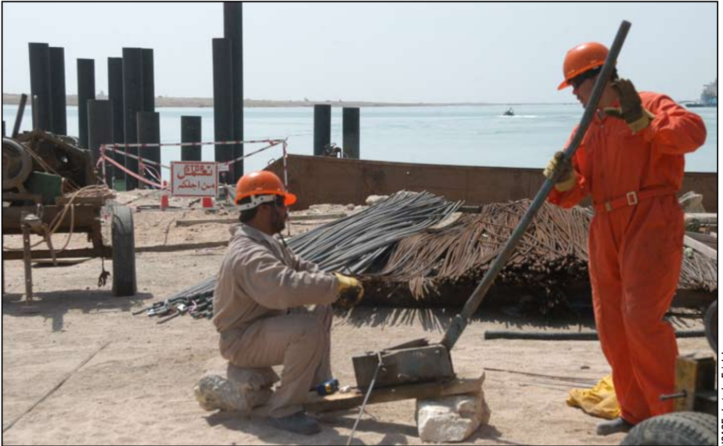
Workers bend reinforcing bar in preparation for concrete placement during construction of the RoRo berth.
