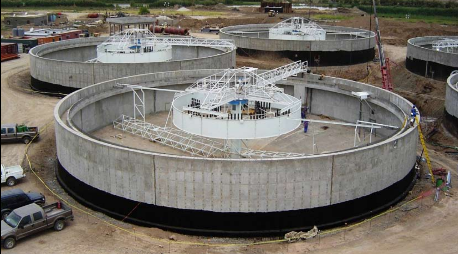
Shown under construction, the volume of the six clarifiers at the Nasiriyah Water Treatment Plant is clear. (USACE photos)
