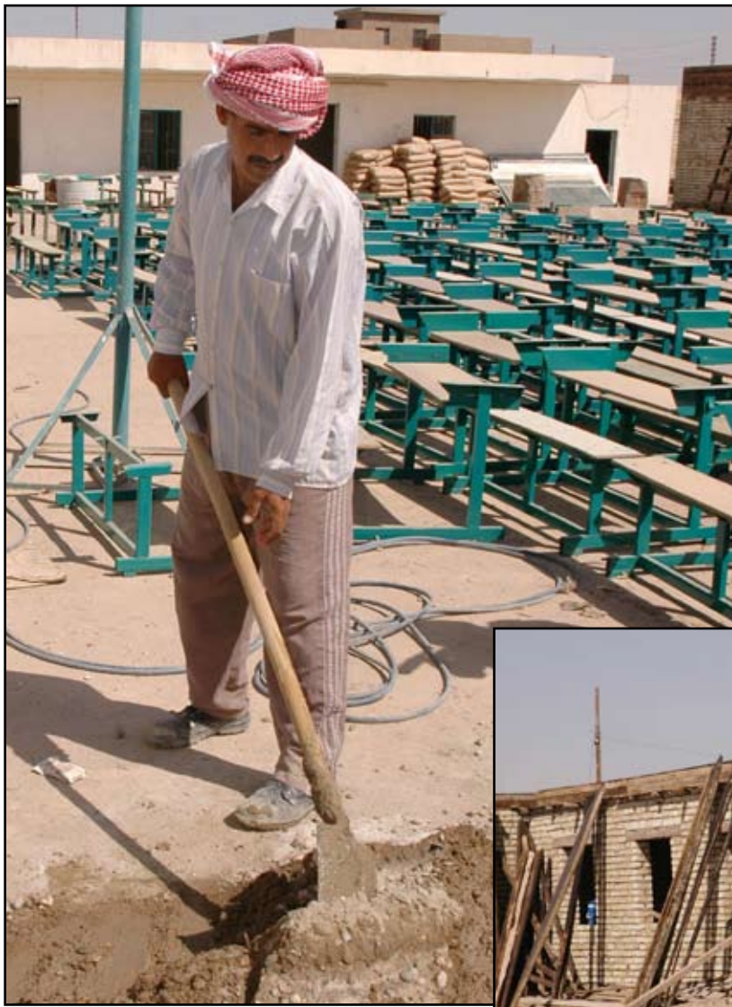
Above: A worker mixes a batch of concrete. Inset: Forms come off after placing a section of the concrete roof.
