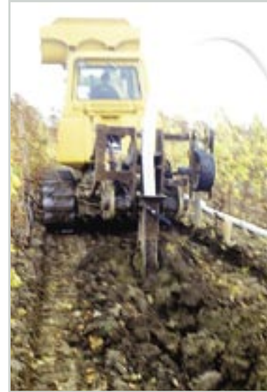
FIGURE 8. Equipment used to install drain tile between rows in a vineyard with imperfect soil drainage. Photos courtesy of Gene Sigel.
