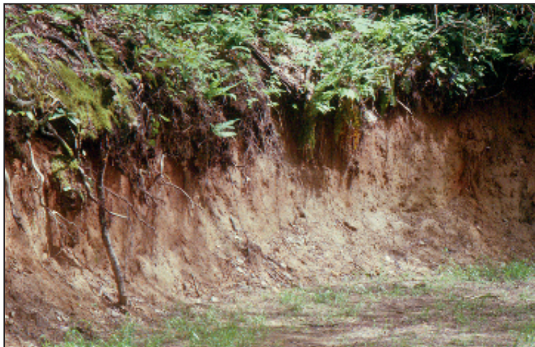
Figure 15. Straight up excavated side cut.
