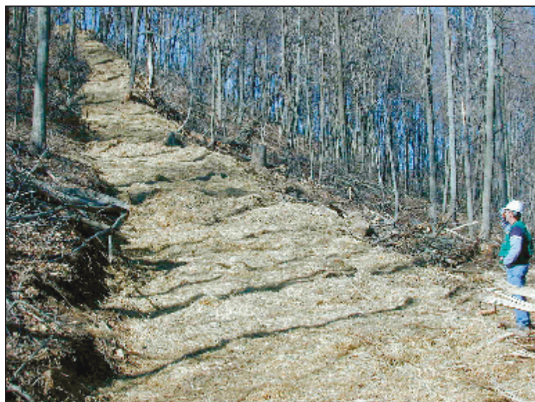
Figure 27. Properly installed mulch on new seeding.
