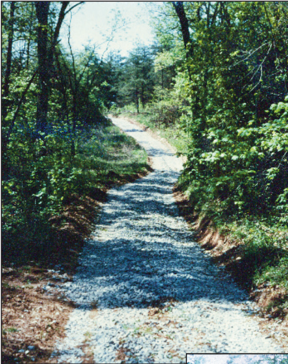
Figure 10A. Broad-based dip examples.
