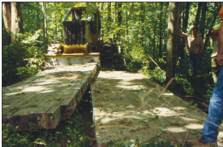
Figure 22A. Portable logging bridge installed with skidder.
