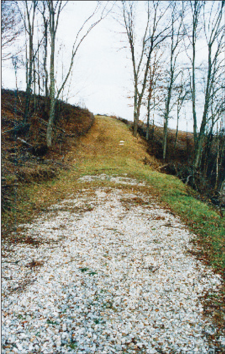
Figure 26. Properly re-vegetated and closed logging road.
