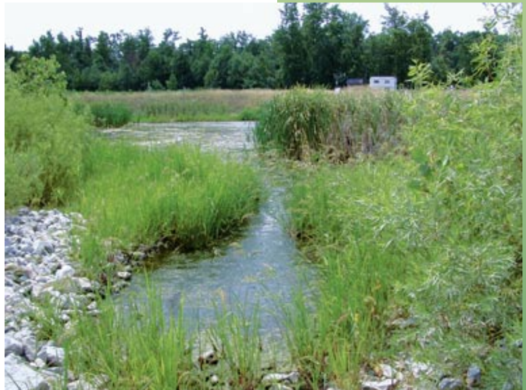
Vegetation growing on “wavy” basin banks at a constructed treatment basin in Defiance County, Ohio.
