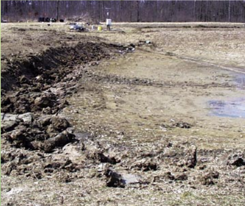
An example of a shelf within a constructed treatment basin in Defiance County, Ohio.
