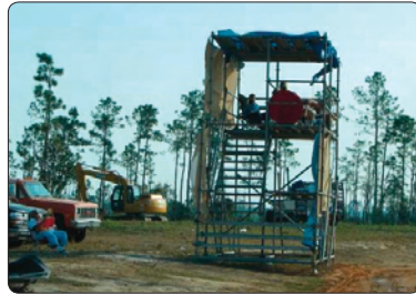
This QA tower is set up to inspect debris trucks going into dumpsites. The inspector is at risk from vehicle traffic traveling near the tower. Notice in this photo, the lack of buffer zone around the tower. There should be visual markings such as cones, signs or tape to identify the tower to the drivers.
