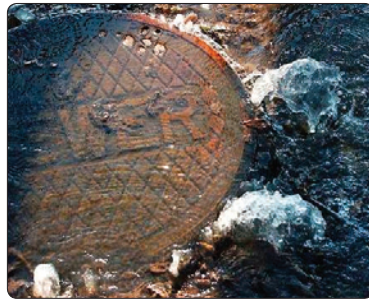
Raw sewage bubbles up from a man-hole cover along U.S. Highway 90 in Gulfport.
