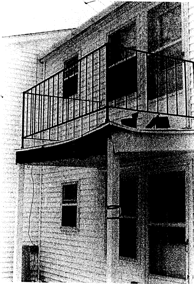
Neglect following from misused funds is clear with this unsafe balcony. OIG photo.
