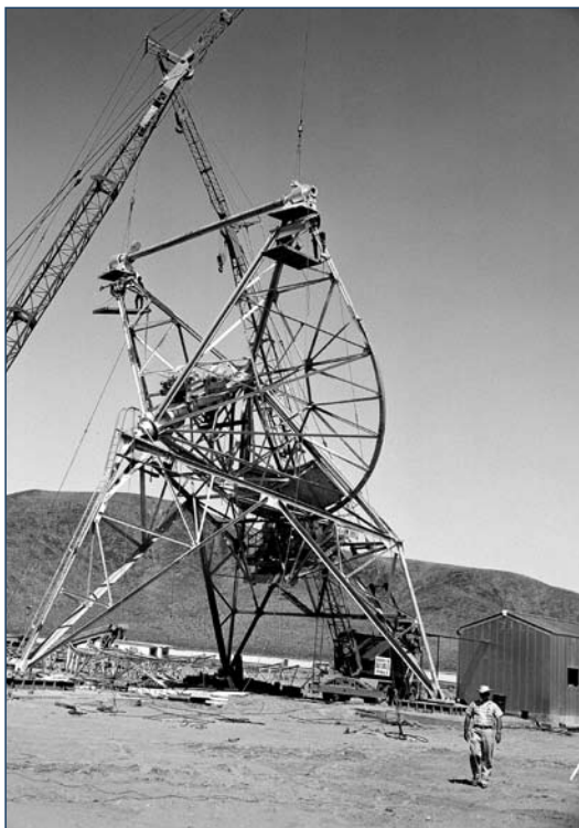
The Pioneer Antenna under construction on 28 August 1958. (JPL File Photo JB1969B)
