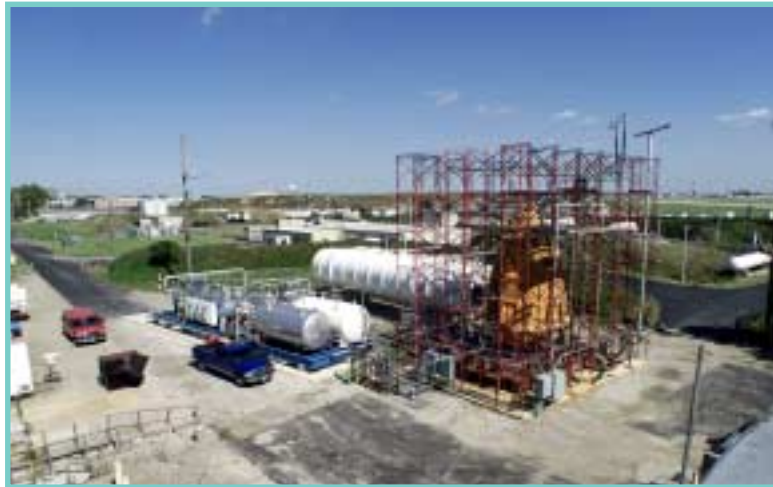
GRC propellant densification test site.
