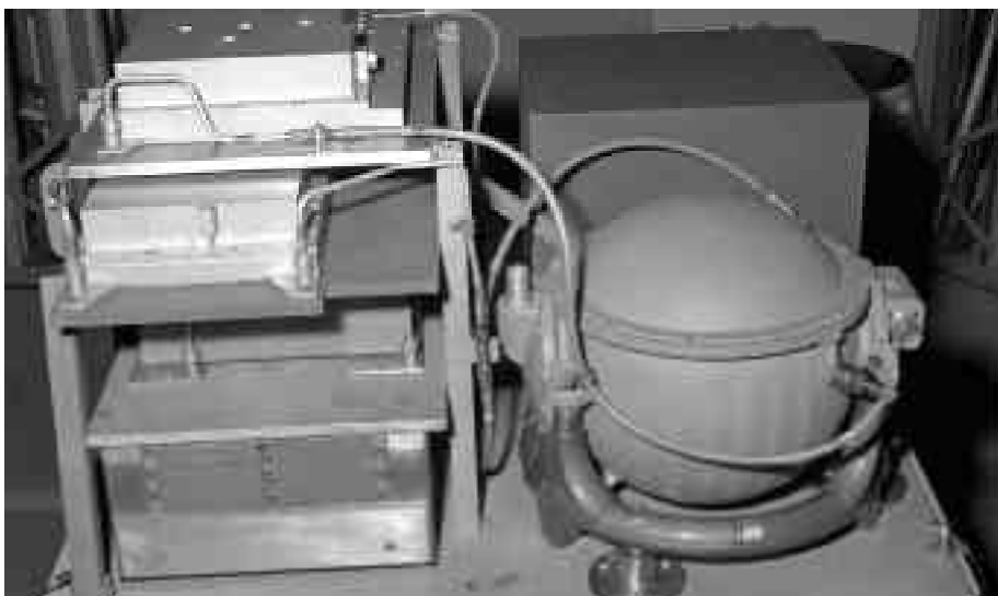
The Apollo guidance computer and the inertial system on a pallet. Note tubing to carry coolant among the cold plates. (NASA photo E-23287).
