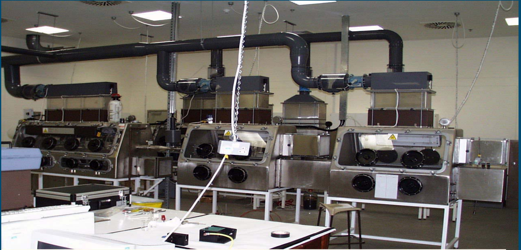
Line 2 - exposure (W9098), generation (W9099) and preparation (W9096) cabinet
