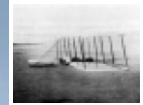
The 1901 Glider: The Wright brothers' 1901 Glider enabled them to spend more time in the air and to uncover additional design problems.
