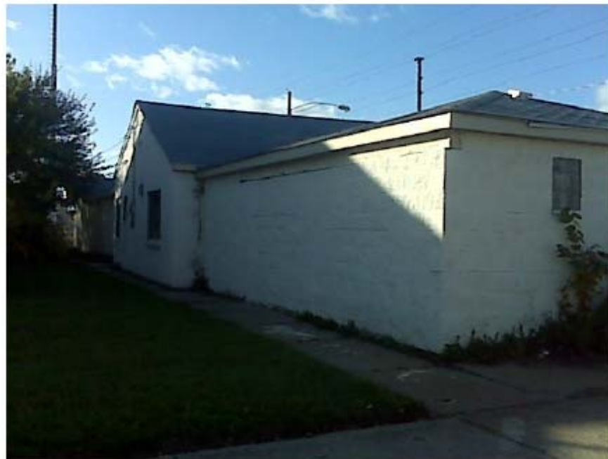
5540 Eight Mile—Rear of Building
