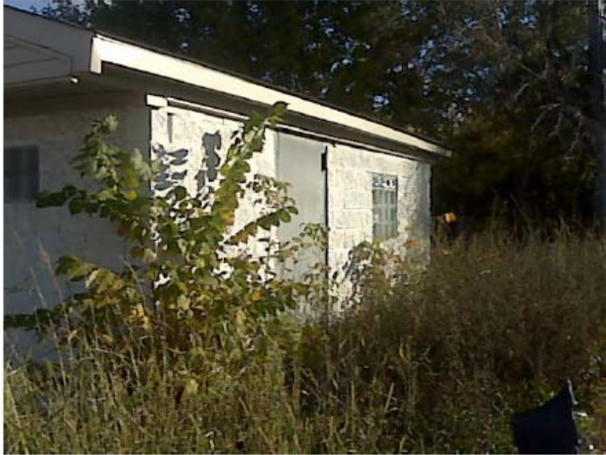
5540 Eight Mile—West Side of Building
