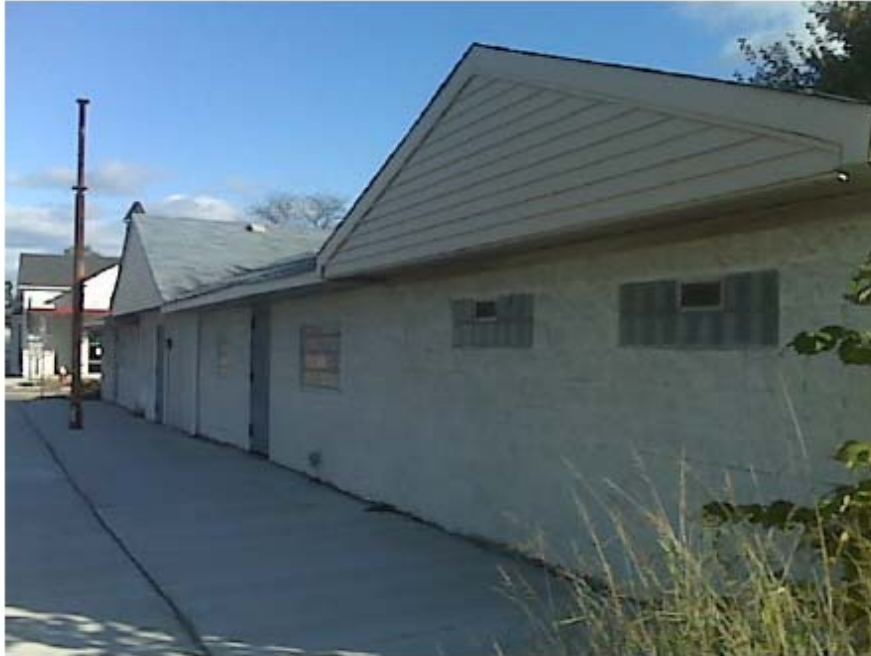
5540 Eight Mile—Front of Building
