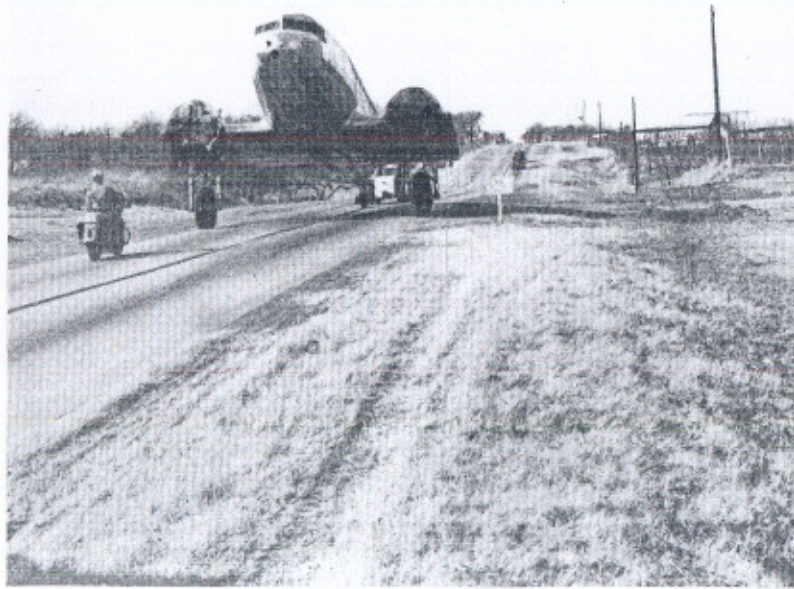
The highways can serve in unusual wartime emergencies. This damaged transport plane, after an emergency landing, was stripped of its wings and towed to the nearest airport.
