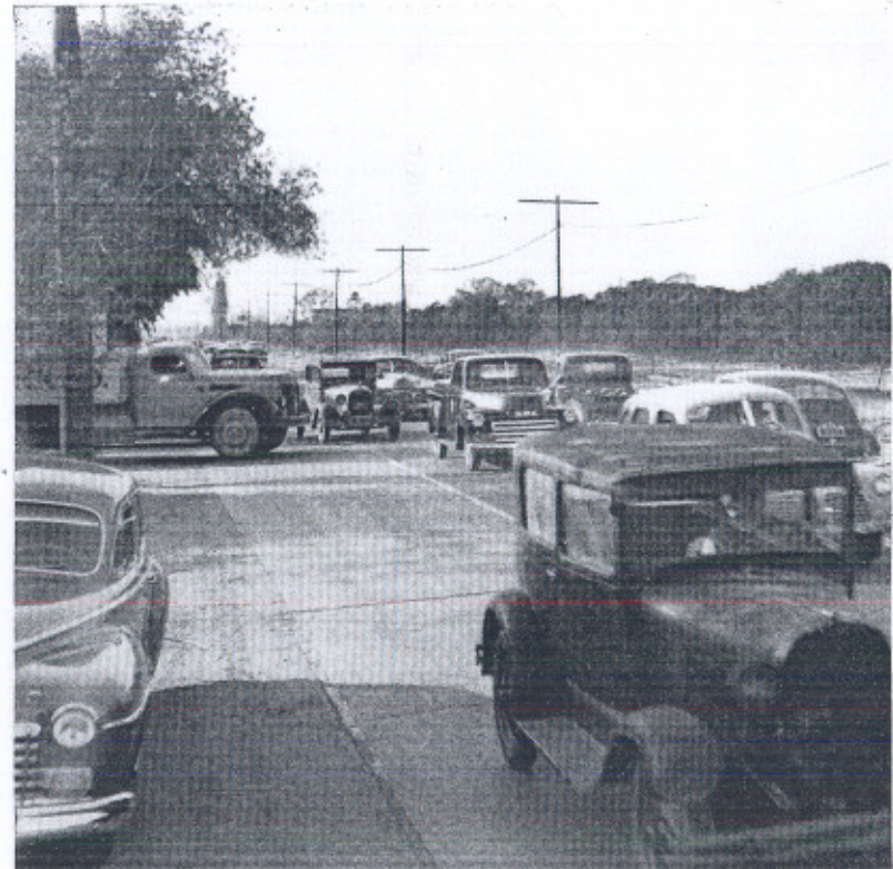
The four-lane undivided pavement on this bypass of U S Route 101 in California was an attempt to cope with mounting traffic volume. The present 20,000 vehicles a day are far beyond the road's practical capacity, and lack of access control prevents free-flowing movement. About 1,350 miles of the interstate system now surfaced with three or more lanes undivided should be rebuilt as multilane divided highways.
