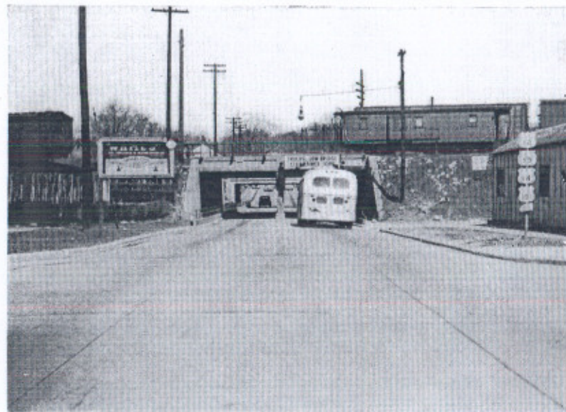
Ten-foot vertical clearance and width narrower than the approach pavement, with the added hazard of a center pier, bottleneck the 13,000 vehicles a day, including 2,700 trucks and busses, that use this underpass on U S Routes 12, 14, and 151 in Wisconsin.
