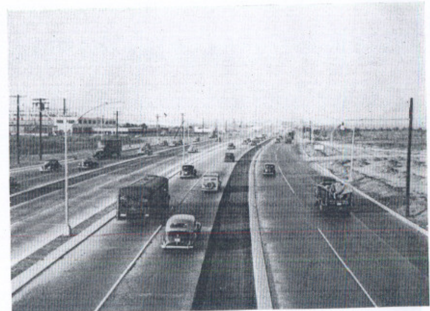
The war proved to be only a temporary interruption to the long-term upward sweep of traffic volumes. This dual-dual section of U S Route 1 near Newark Airport, New Jersey, now carries about 70,000 vehicles a day.
