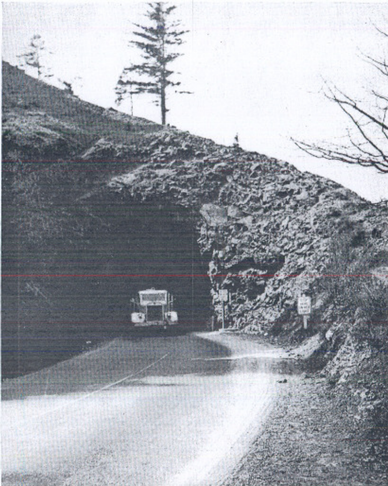
The Mitchell Point tunnel on U S Route 30 in Oregon is so narrow, and its approaches so winding, that traffic-actuated signals were installed to operate the tunnel one way alternately in either direction. Every tunnel on the interstate system is in some degree inadequate in horizontal clearance.
