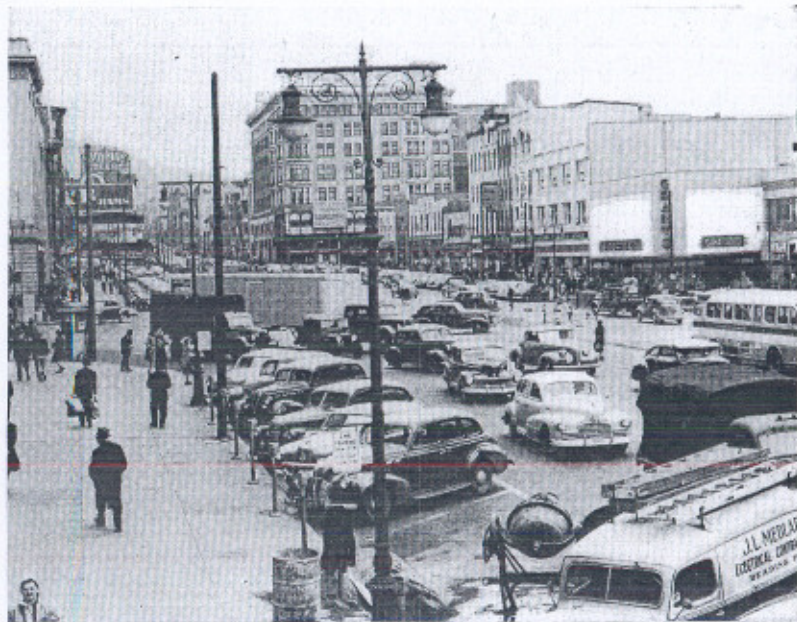
This street is U S Route 422 in Reading, Pa. Its extreme width is negated by the lack of channelization or control, as evidenced by the haphazard, crowded vehicular movements.
