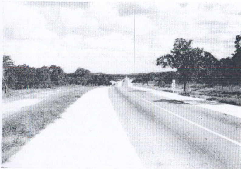
More than 71 percent of the rural mileage of the interstate system—22,684 miles—is without 8-foot minimum width shoulders, such as these on U S Route 87 in Texas.
