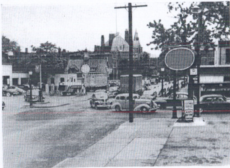
Free flow of traffic and turning movements on urban portions of the interstate system are often hampered by traffic lights, narrow streets, parking, and entrances to gasoline stations and other business establishments, as shown here on U S Route 1 in Virginia. Improvement to interstate system standards would save 21 billion vehicle-minutes—almost 40,000 years—annually.
