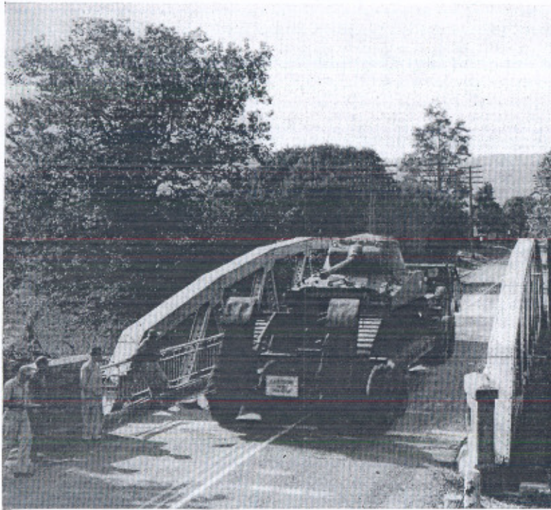
This bridge on U S Route 30 in Pennsylvania, designed for about H20 loading, is strong enough to carry infrequent loads as heavy as the 152,000-pound tank transporter and tank. For adequacy, the bridge should be wider than the approach pavements.
