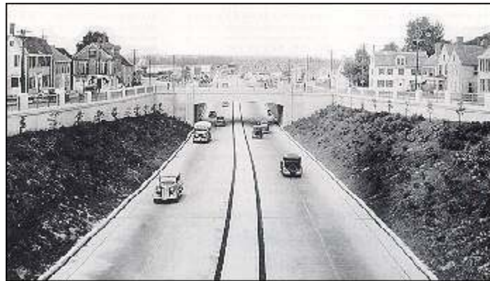
Early freeway in Newton, Mass., circa 1935, showing access control.
