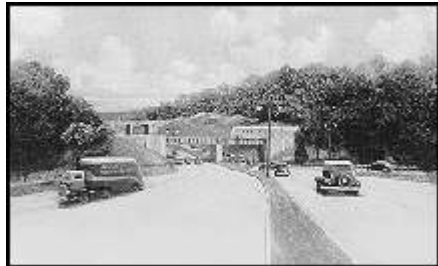
Model of a six-lane divided highway shown at the New York World's Fair in 1939 to illustrate the method of making highways safer by separating both railroad and highway grade crossings.
