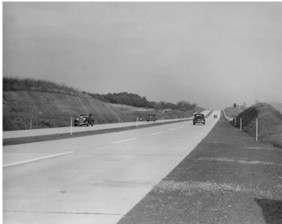
Design of the Interstate System evolved from earlier freeways, such as the Pennsylvania Turnpike (above) and the Arroyo Seco Parkway (below, now the Pasadena Freeway) in Los Angeles, both of which opened in 1940.
