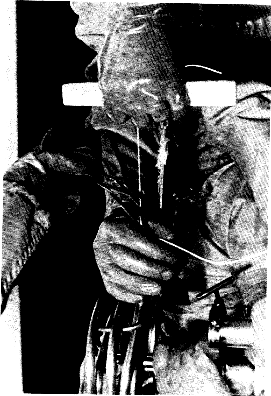
Figure C4-40.- Pulling first bundle of heater and fan motor leads into upper coil assembly.
