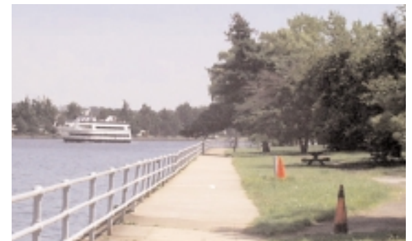
Washington Channel shoreline provides an appropriate landscape setting for a future commemorative feature that would reflect the park-land context of East Potomac Park's waterfront
