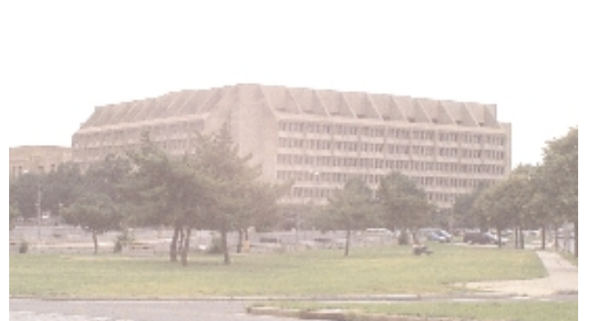
View looking west toward HHS building from Washington Avenue where potential commemorative features could be located within existing public spaces near the Mall
