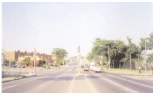
The view above looks northeast on New York Avenue with the bridge over the rail lines in the background. Potential memorial sites are located on both sides of New York Avenue. The potential redesign of the intersection would influence future site opportunities.
