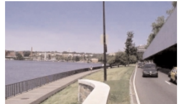
This site offers potential for future memorial elements that could reinforce the waterfront setting within a proposed stairway connection from the Center's terrace to the river edge
