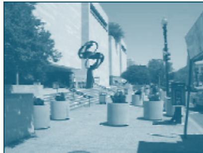
Existing temporary security measures at the National Air and Space Museum
