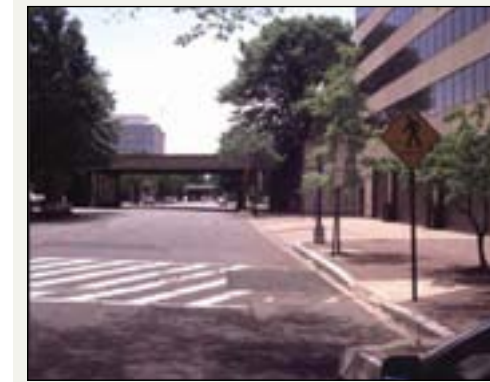
6th Street, SW, looking south
