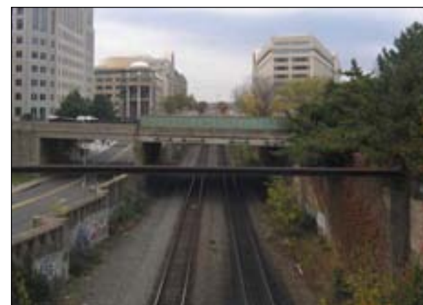
Existing rail line within the Maryland Avenue right-of-way looking west
