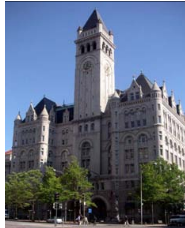
The Old Post Office building garners a commanding presence along America's Main street
