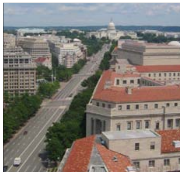
With its limestone facades, red-tile hipped roofs, and classically inspired colonnades the Federal Triangle is a fine example of public architecture.
