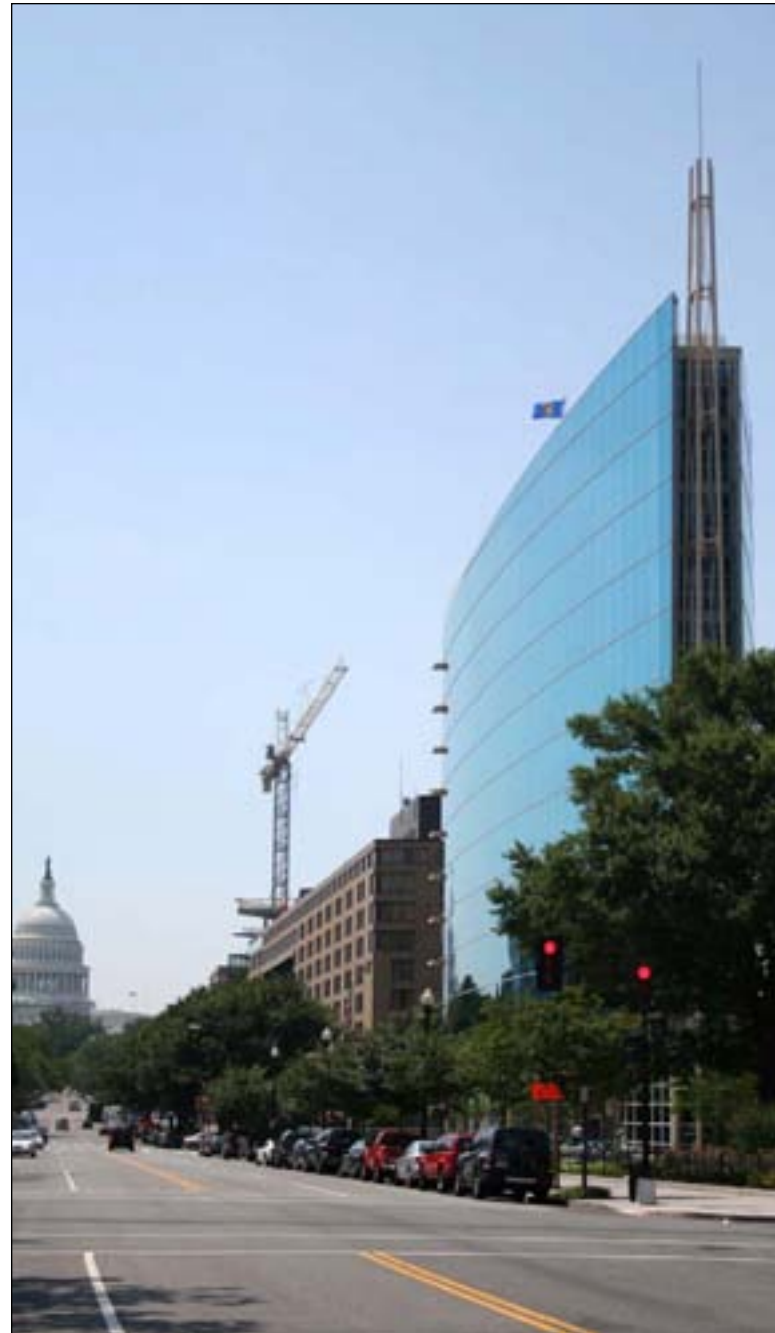
The National Association of REALTORS building incorporates many environmentally sustainable features.
