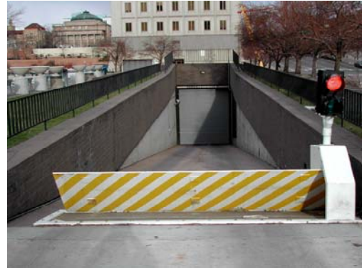
Vehicle barriers such as this and other access control measures assist in managing vehicles approaching a submerged access point.
