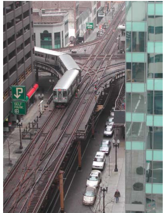
Elevated structures might span unusual natural features or navigate dense development.
