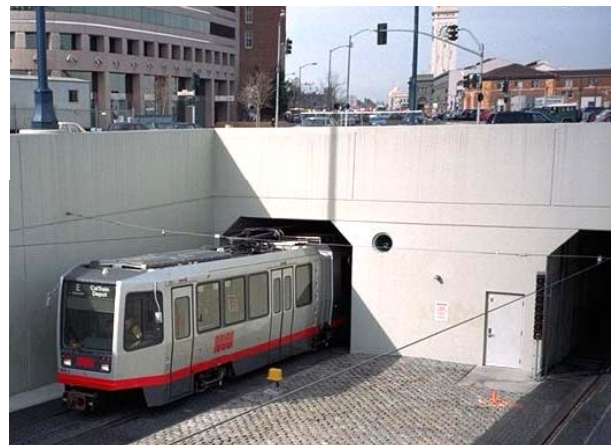
Fencing and a grade change help segregate this portal from nearby public areas.
