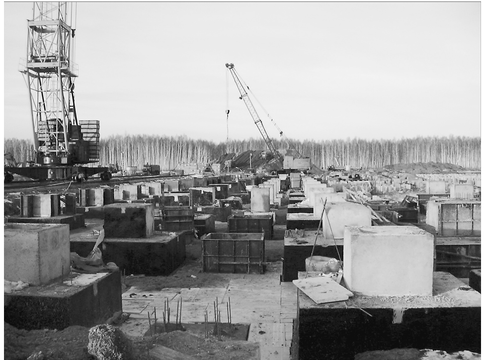
Figure 5: Construction of the Russian Destruction Building at Shchuch'ye, November 2003
