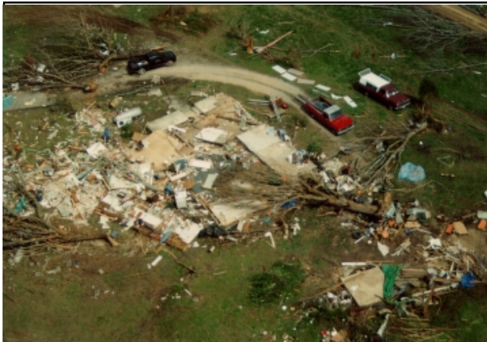
F4 to F5 damage occurred in F3 intensity winds as house was not anchored to its foundation. Photograph courtesy of _____.
