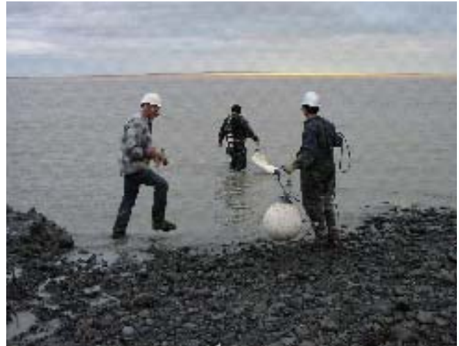
A diver wades into the Nushagak River to plug the end of the sewer outfall.
