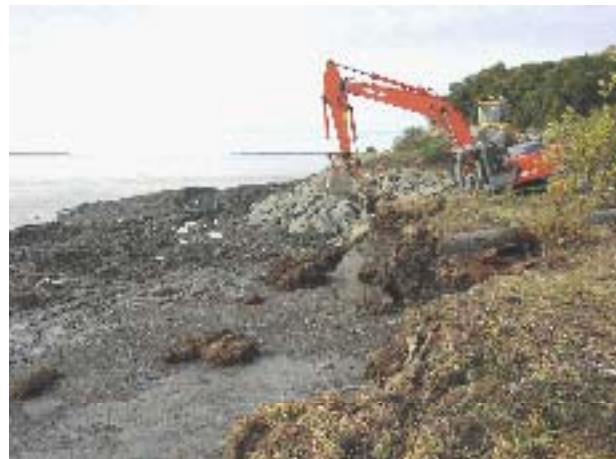
Tying the project into the eroded upstream bank.
