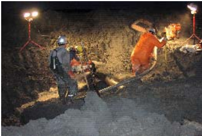
Work continues through the night to replace the sewer outfall.
