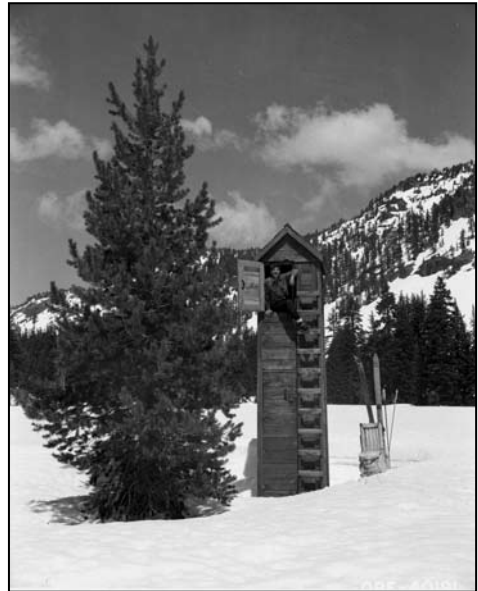
4.5 Arch Work on a Santa Claus chimney entrance, Crater Lake National Park, 1945
