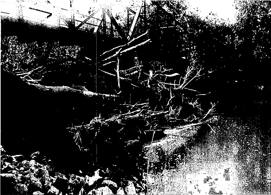
Debris blocks a bridge near Hannibal, Missouri. Under the Emergency Watershed Protection program, SCS contracted to remove this obstruction. Photo by author.
