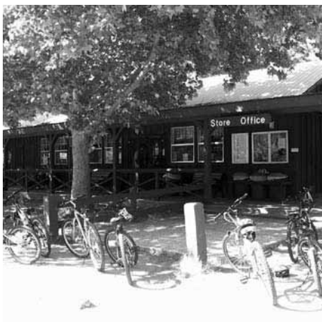
Campground store and visitor center.
