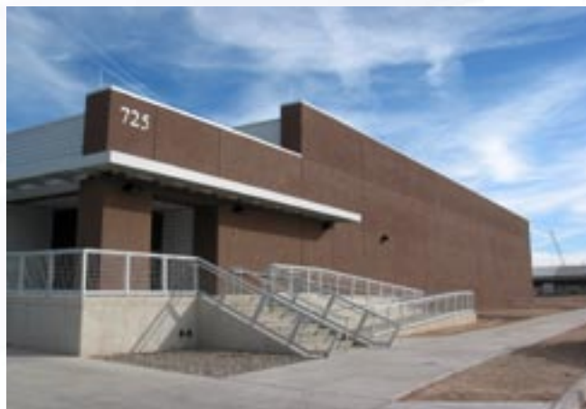
The home of Red Storm, The Supercomputing Annex at Sandia National Laboratories.
