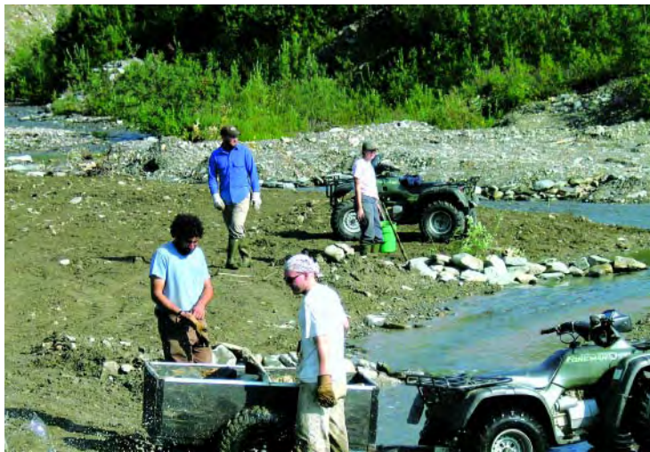
Glen Creek Crew rebuilding stream channel
