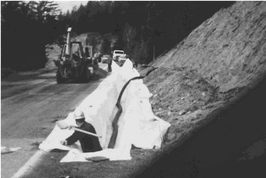
Figure 67. Photo. Installation of longitudinal drainage to reduce frost heaving.
