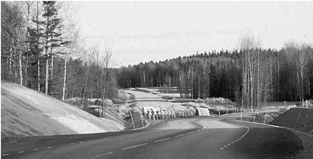
Figure 66. Photo. Road construction in Sweden with deep base section.
