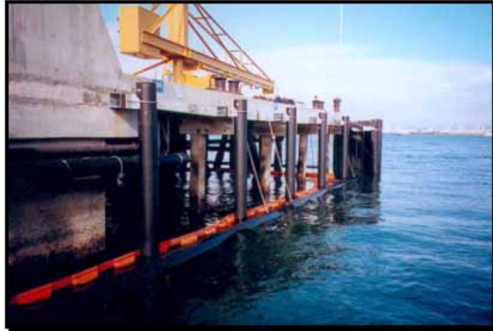
Figure 3. Photo. Fender piles in the U.S. Naval Submarine Base, San Diego, CA.
