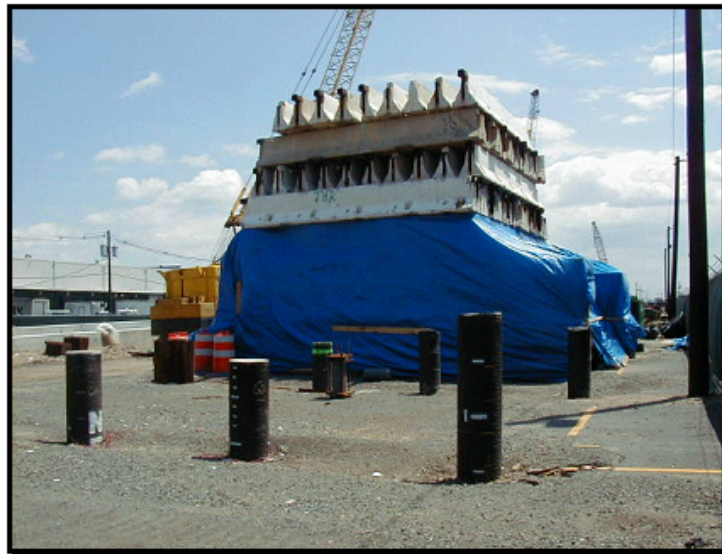
Figure 7. Photo. Port of Elizabeth demonstration site.
