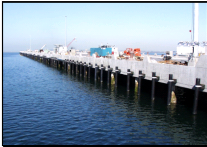
Figure 4. Photo. Fendering system in the U.S. Navy Pier 10, San Diego, CA.
