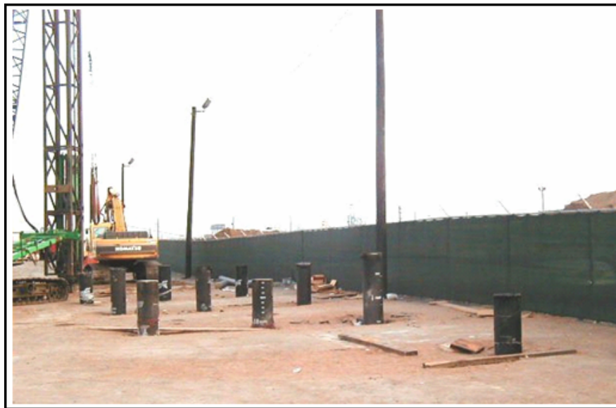
Figure 39. Photo. Port of Elizabeth demonstration site.
