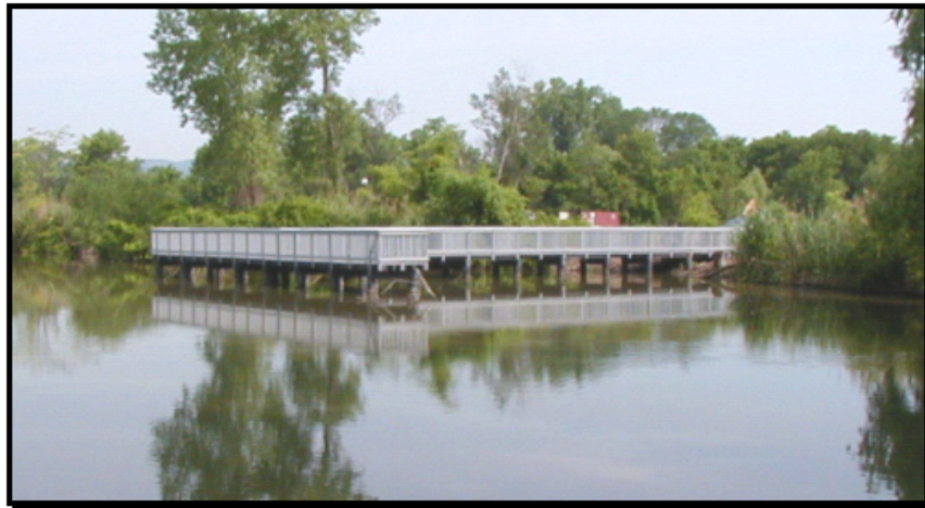
Figure 6. Photo. Floating dock project.
