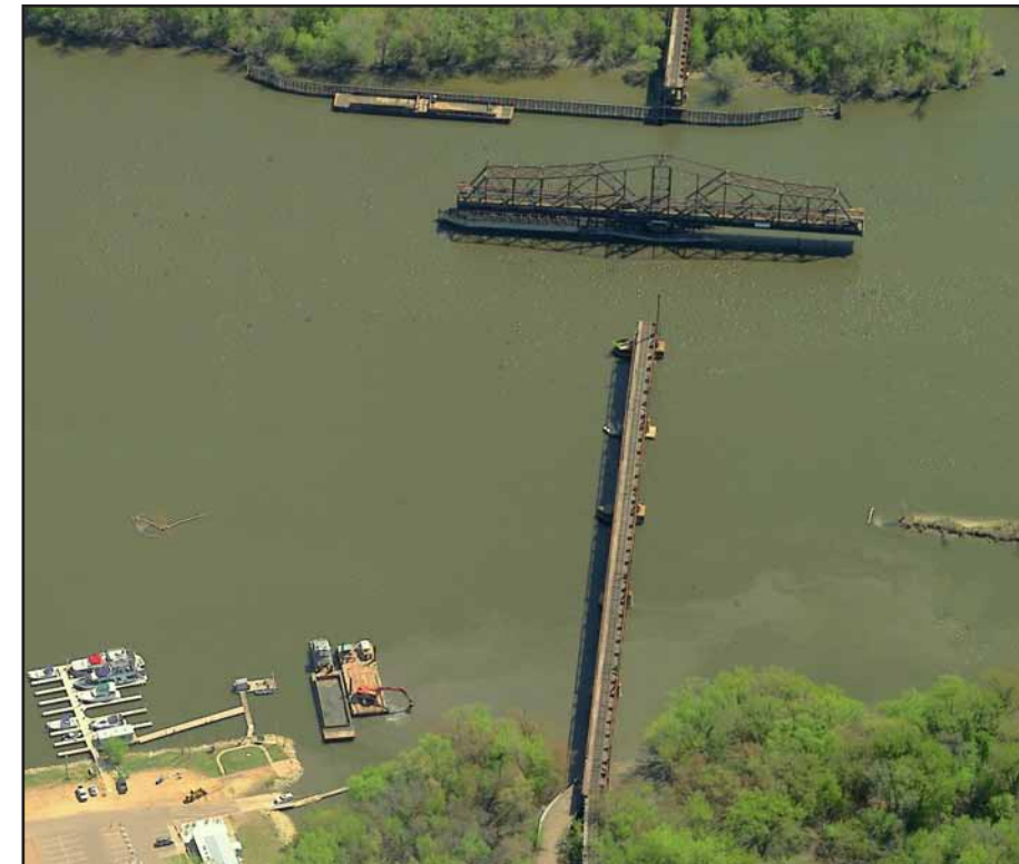
Looking east, toward Washington County side
