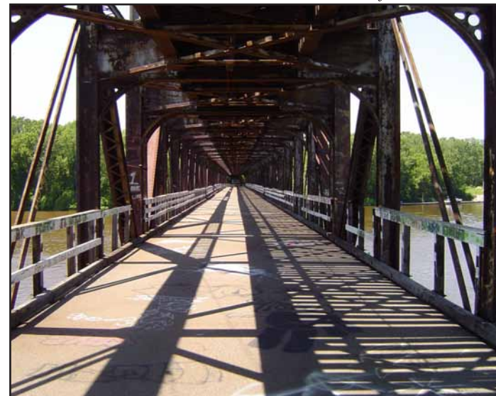
View from lower deck
