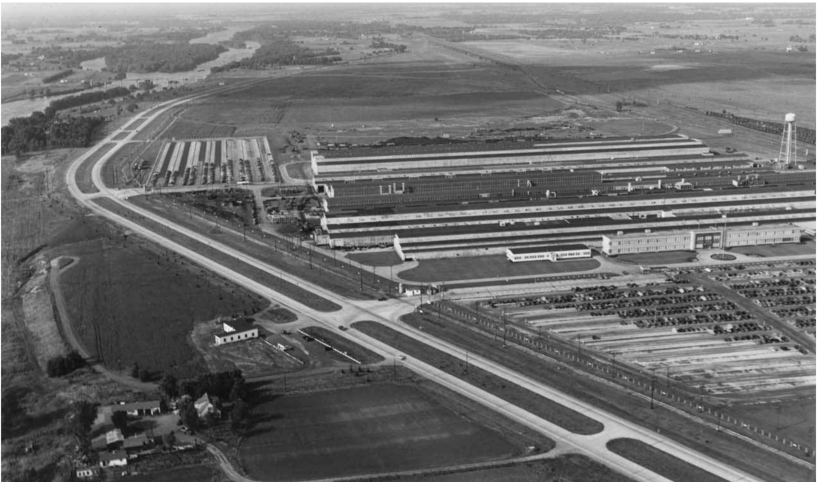
FIGURE 8. East River Road, Fridley, 1945. The Northern Pump Company is the large building complex. Minneapolis Star Journal Tribune Photograph, Minnesota Historical Society.
