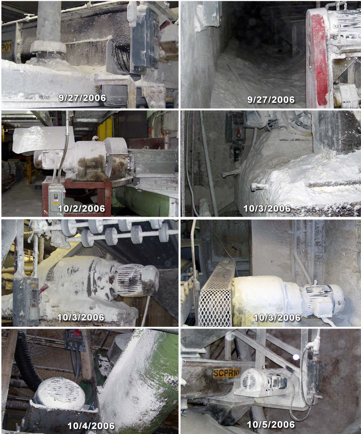
Figure 3. Photographs of sugar accumulations inside the Imperial Sugar Port Wentworth facility from September – October 2006.
