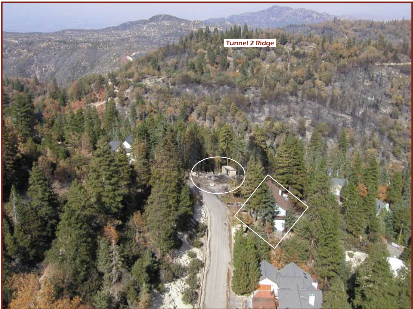
Figure 31. Aerial view looking northwest up Walnut Hills Dr. to destroyed home at 26142 (circled) and damaged home at 26150 (framed). Tunnel 2 Ridge is directly across drainage and shows evidence of group tree torching.
