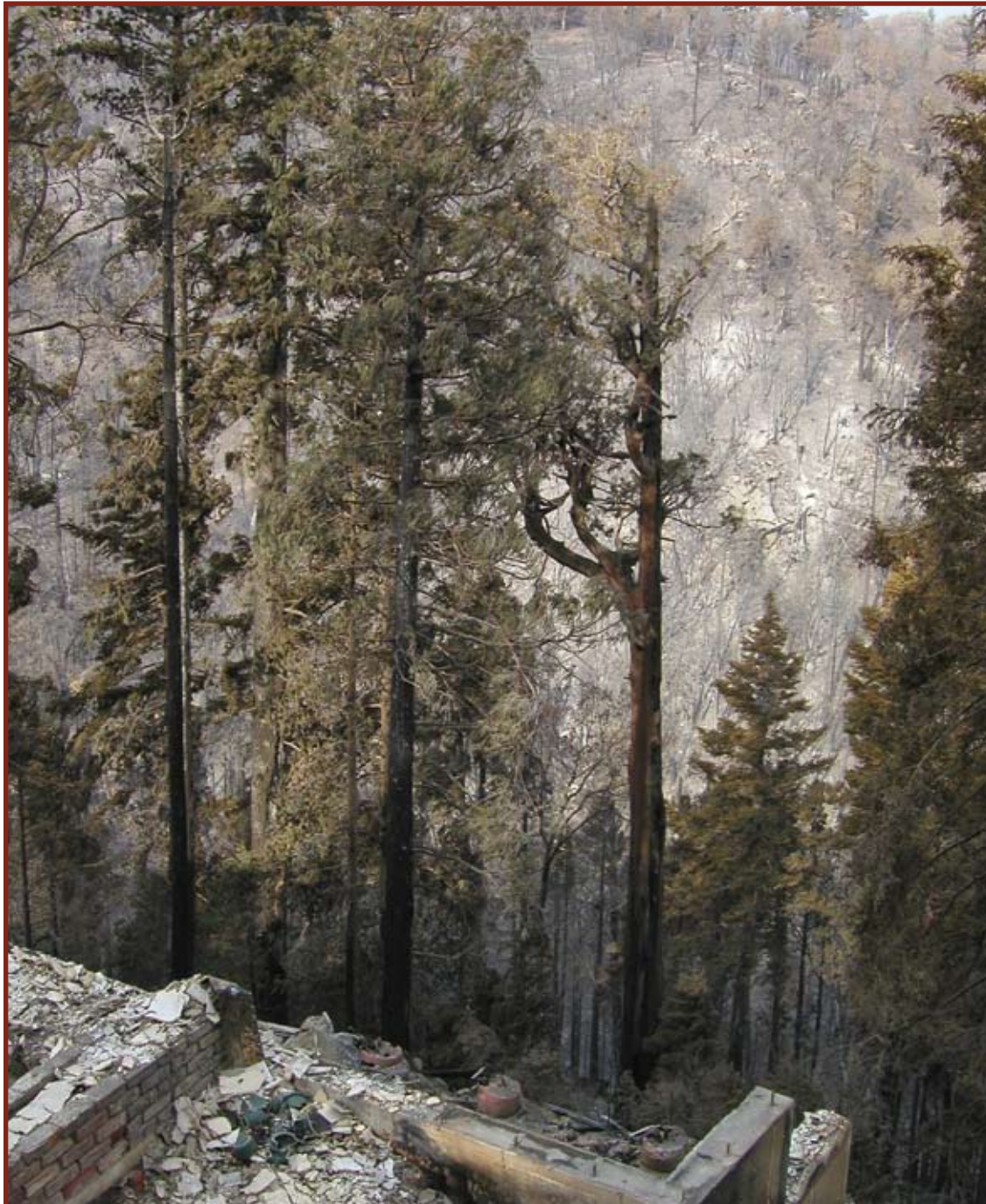
Figure 13. Destroyed home at 1114 Brentwood Dr. looking across Grass Valley drainage west. Note the unconsumed canopy indicating this home was destroyed by surface fire and/or directly ignited from firebrands.
