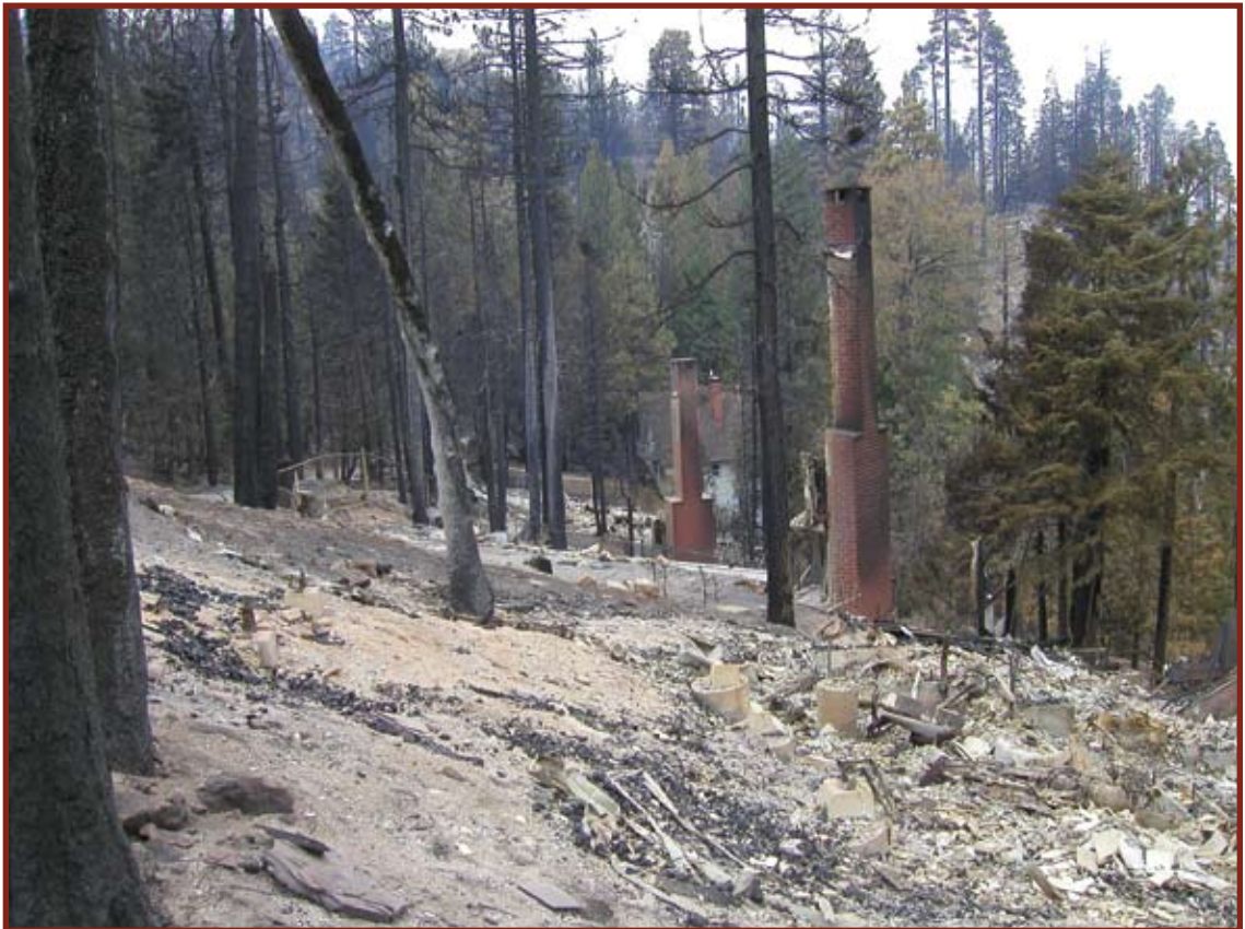
Figure 25. Four destroyed homes on Brentwood Dr. looking northwest. The home in the background is 850 Brentwood.
