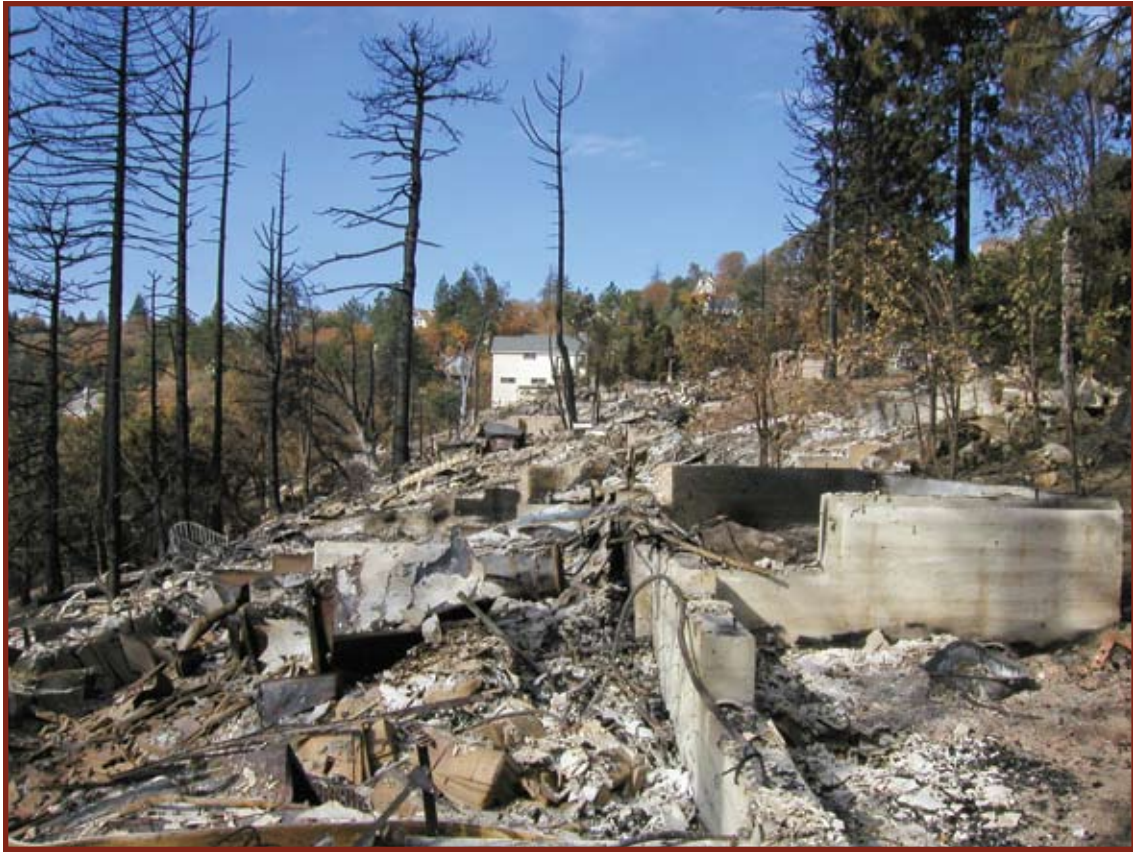
Figure 26. View looking west through seven destroyed homes on Merced Ln. to the white house at 26665.
