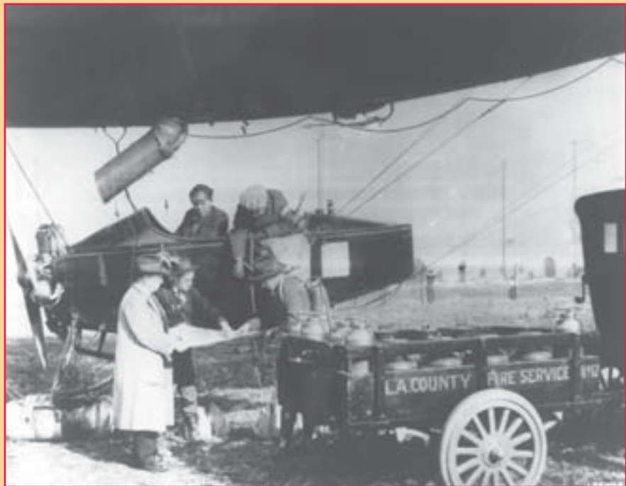
Blimp tested for fire patrol on the Angeles National Forest, CA. The carriage suspended from the balloon (visible at top) could carry firefighters, supplies, and equipment. Photo: Courtesy of National Agricultural Library, Special Collections, Forest Service Photograph Collection, Beltsville, MD (W.I. Hutchinson, 1921; 156936).
