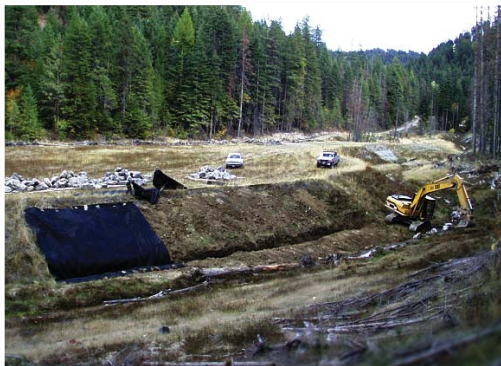
Reclamation work underway at the Cleveland Mine site in Washington.
