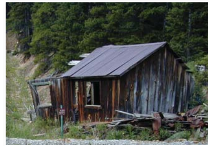
A former mining structure near the Elk Tunnel Mill in Colorado.
