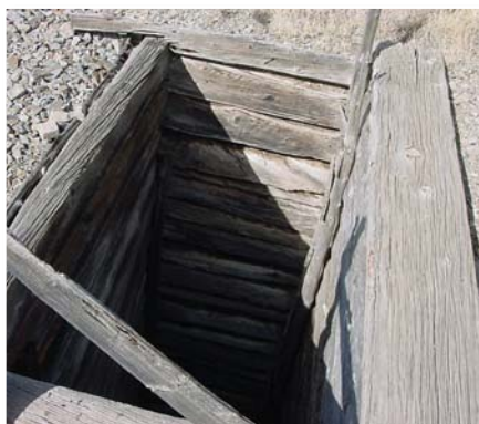
One of several open vertical shafts addressed at the Reef Gulch site in Colorado.
