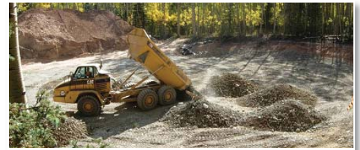
Waste rock from the Buffalo Mine in New Mexico being dumped in the repository.
