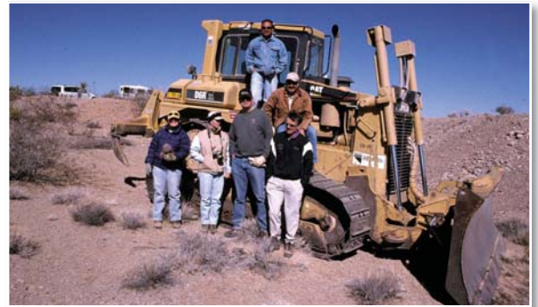
Members of the 2005 backfill team in Southern Nevada during a week of intense AML shaft backfilling.
