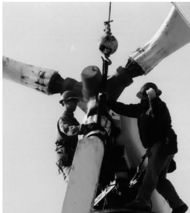
Figure 5. 7 Photographs of the Rotor Blade Installation
