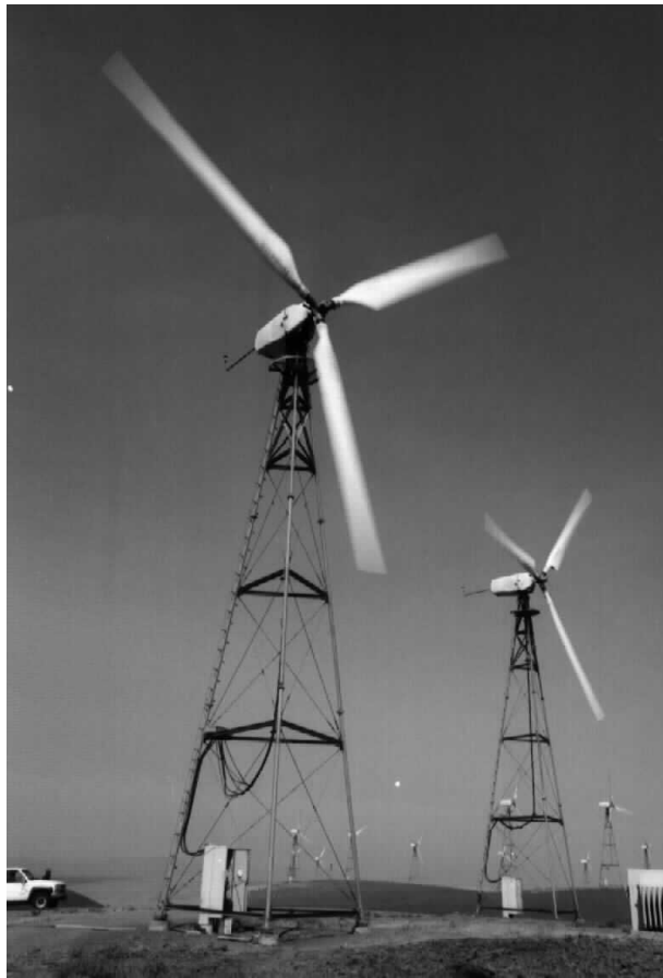
Figure 5. 1 Photograph of the Two Operational Test Turbines
