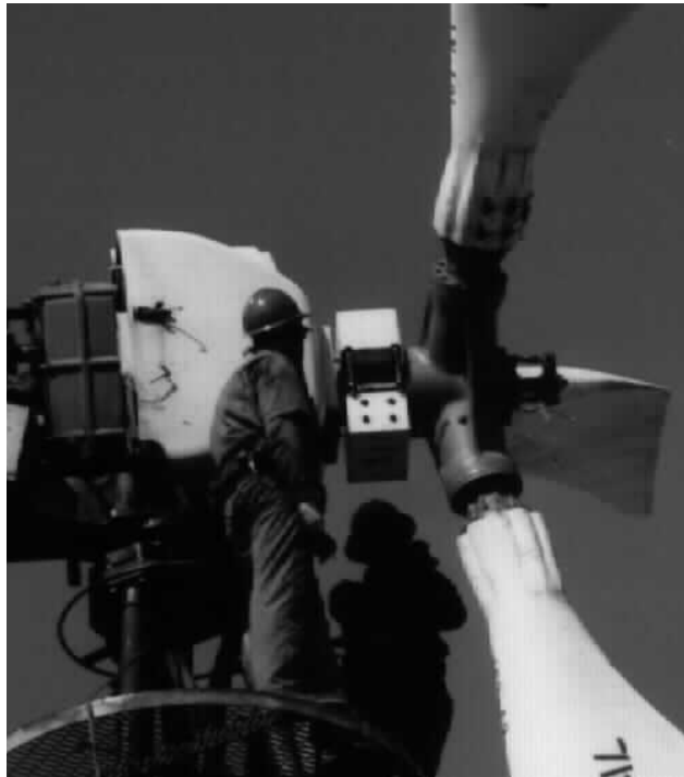
Figure 5. 8 Photograph of the Rotor Instrumentation
