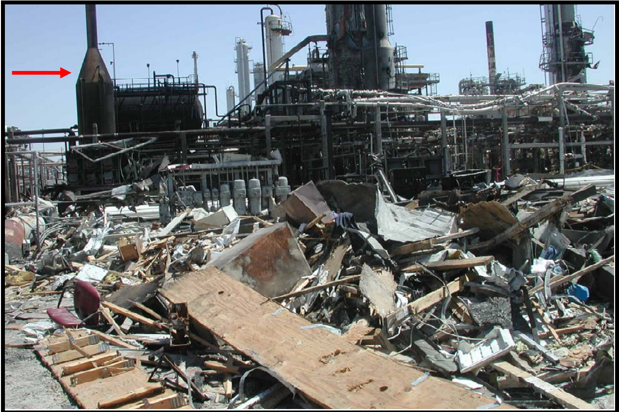
Figure 13. Destroyed trailers west of the blowdown drum (red arrow in upper left of the figure)
