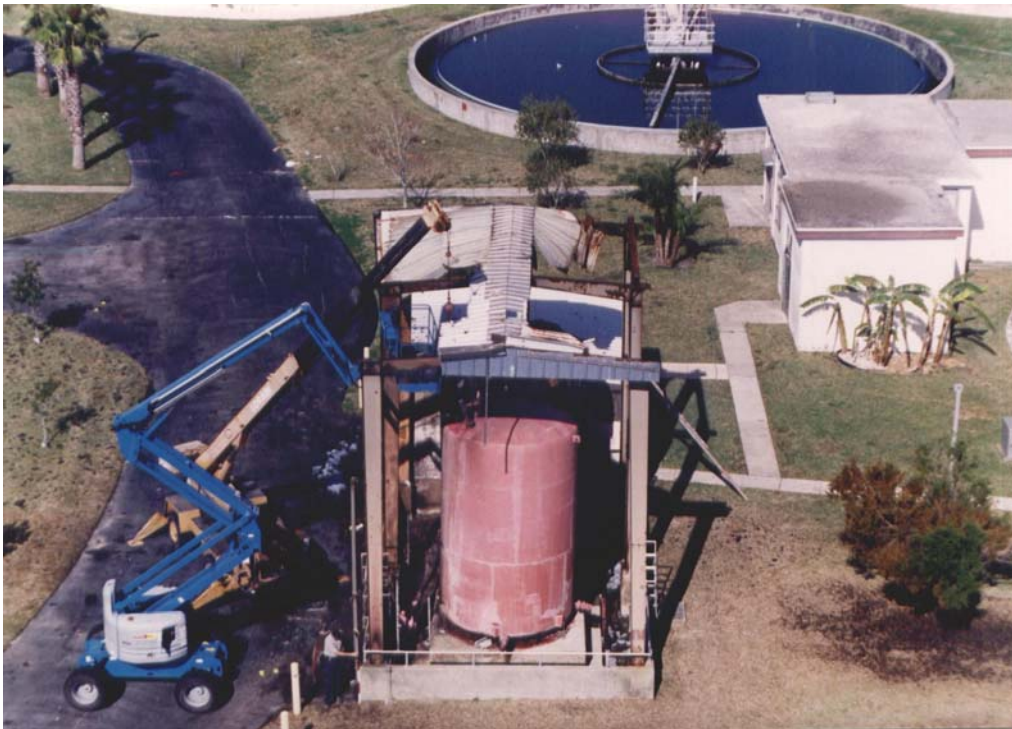
Figure 2. Bethune Point WWTP accident site.
