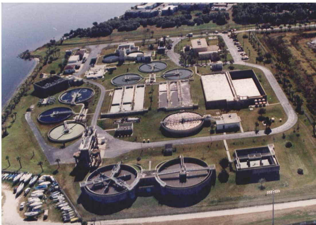
Figure 1. Bethune Point WWTP. (Picture courtesy of the City of Daytona Beach)
