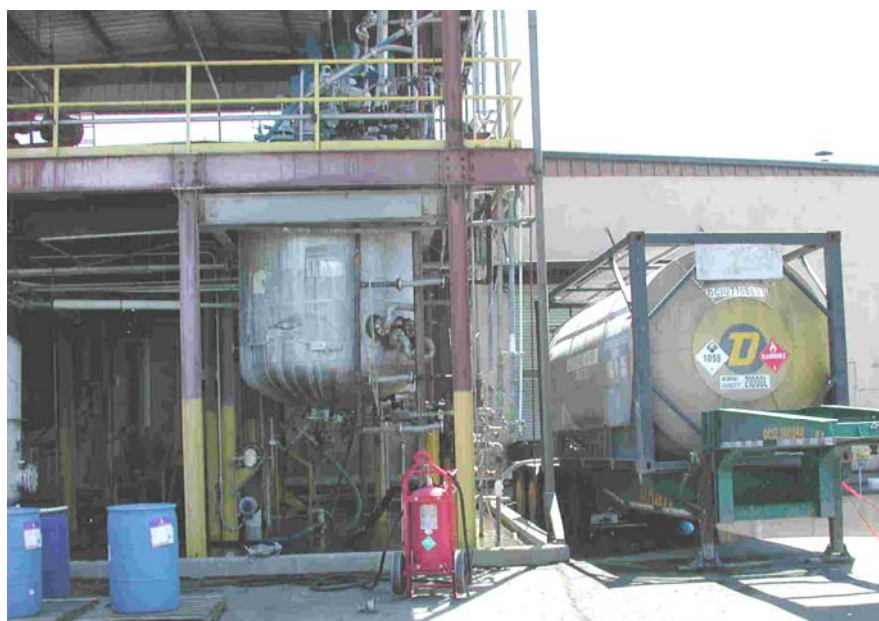
Figure 7. Isotainer (right) positioned adjacent to the process equipment.
